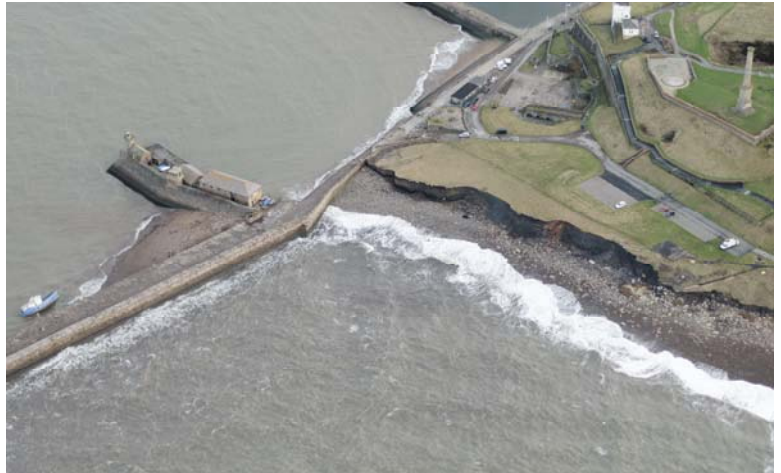
Erosion to the coastline adjoining Whitehaven harbour. The harbour walls were also damaged during the event.
